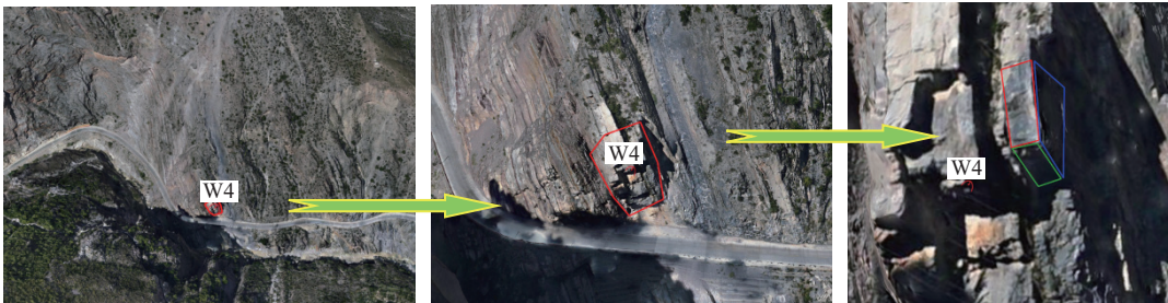
图 10 W4 崩塌体结构面全局-细节图 Fig. 10 Global-detailed view of the structural surface of the W4 collapse body
