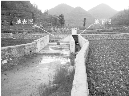
图 3 陈旗岩溶泉系统排泄区的地表、地下复合堰 Fig.3 Compound weirs of surface and underground water in discharge area of Chenqi karst spring
